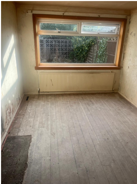
A stripped room showing the starting condition.
