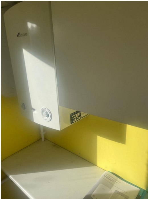
Existing services reviewed as part of the wider upgrade.
