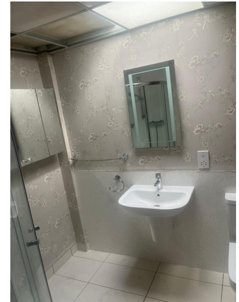
Existing bathroom finishes due for replacement.
