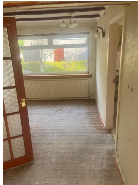
Dated internal spaces ready for full refurbishment.
