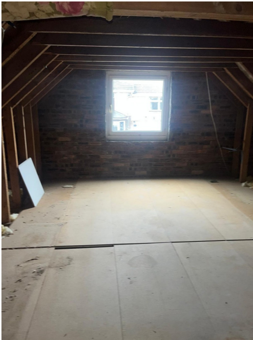
The original roof space before the main conversion works.
