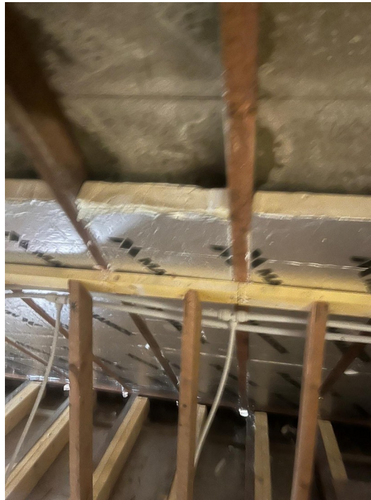
New structural members coordinated around the existing fabric.
