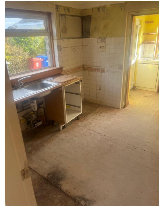
The original kitchen taken back for replacement.
