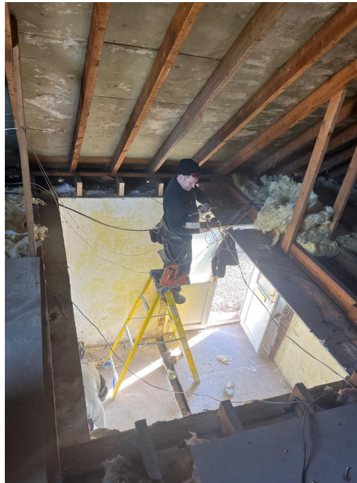
Insulation and lining works progressing through the roof slopes.
