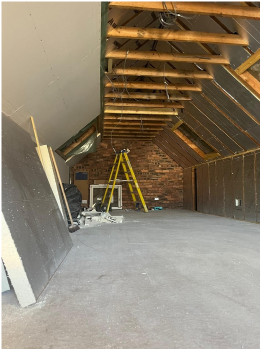
Upper rooms prepared through the finishing stages.
