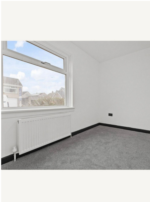
A completed bedroom with new finishes and heating.
