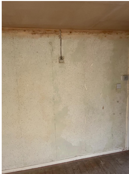
Wall finishes removed to expose the existing substrate.
