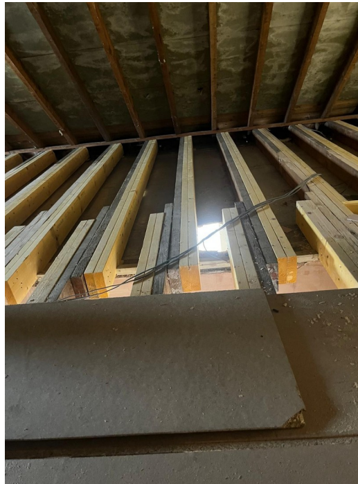
Open construction allowed new routes to be coordinated before closing up.
