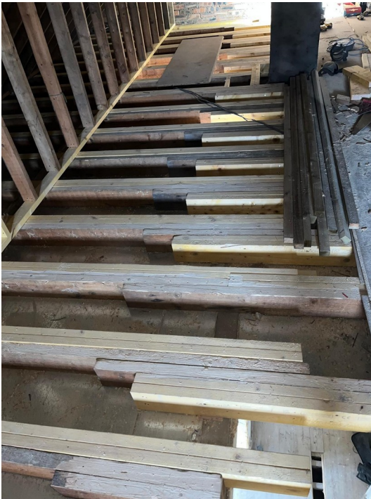
Existing floor structure opened for inspection and strengthening.
